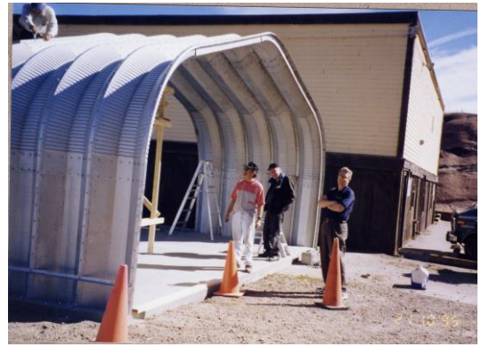
Optimists erecting the Quonset hut
