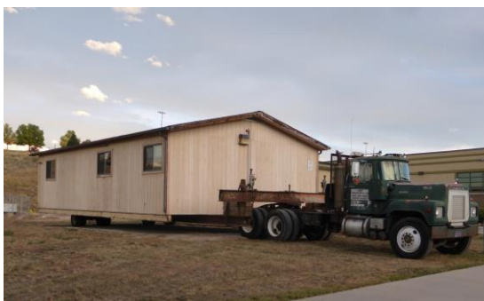
Installing the new temp building at CLC
